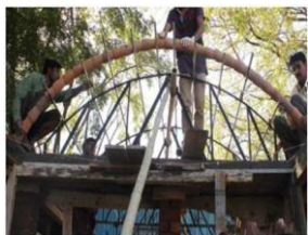
Fig 17 Laying of Guna Tiles
