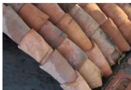
Fig 19. Tying of Guna Tiles Laying
