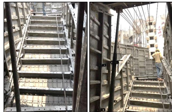
Image 4. - Staircase reinforcement and panel support
