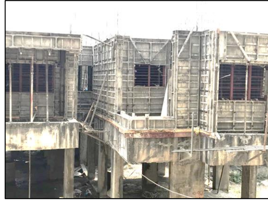
Image 3. - MIVAN construction EWS building
