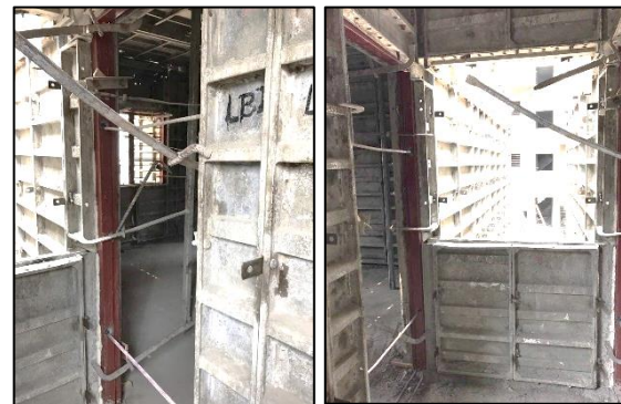
Image 4. - Staircase reinforcement and panel support
