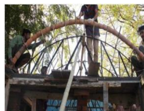
Fig 17 Laying of Guna Tiles Fig 18 Section showing
