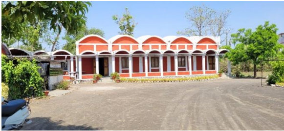
Fig 30 Wardha Block House
