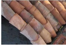
Fig 19. Tying of Guna Tiles Laying
