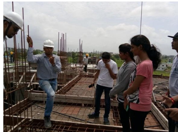
Fig.4) Field trip before laying of concrete for slab, Pune
