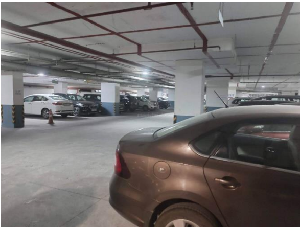
Fig: 14 parking space
