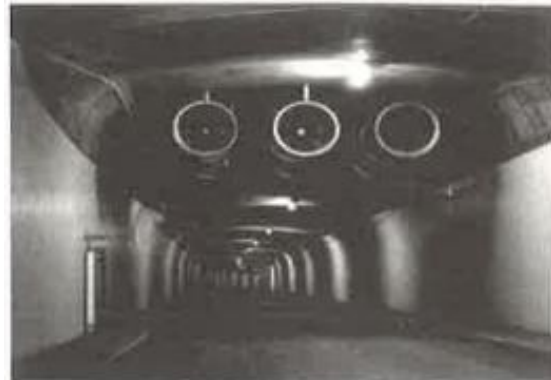
Fig: 4 Ductless Ventilation System
