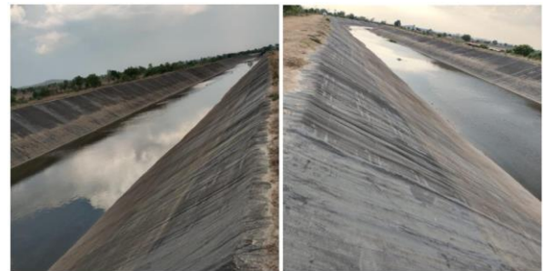
Fig 5: Condition of Canal in January, 2023
