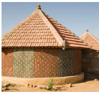
Fig. 6 Coursed rubble masonry, Stone wall Bhunga
