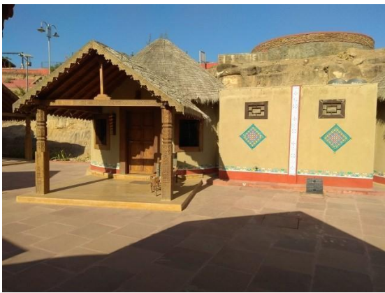
Fig. 4 Mud wall Bhunga house Location: Regenta Resort, Bhuj
