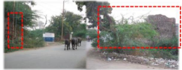
Fig 5:- Condition of Fortified wall
