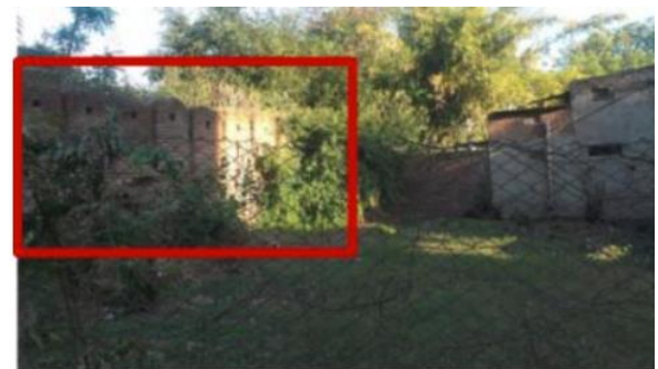
Fig 6:- Condition of Fortified wall
